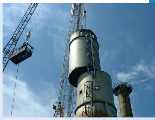
basket nearly 350 feet in the air to allow crew members to perform rigging and dismantling of the stack and breeching. The project was complicated by the close proximity of live power lines, cooling towers, and the new power-house, which was required to remain online for the duration of the project.
