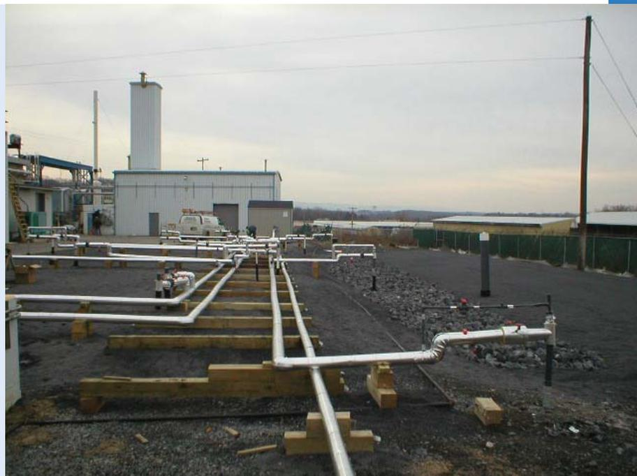
In cases where contaminants lie below the water table, a process called air sparging is used in tandem with SVE. Injection wells are drilled to a level beneath the water table and an air compressor pumps air through the wells into the groundwater-soaked soil. This causes vapor-laden air to bubble up through the groundwater and into the soil above the water table, where it is extracted using SVE.
