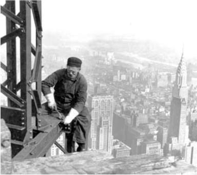
Construction of the skyscraper was a marvel of efficiency. Production, transport and construction were choreographed to a science. Steel girders produced in Pittsburgh, PA were erected and riveted in as little as 80 hours from the time they rolled from the furnaces. Roughly 10 million bricks and 200,000 cubic feet of Indiana limestone were used. More than 3,400 workers, including hundreds of Mohawk Indian ironworkers, took part in the project.
