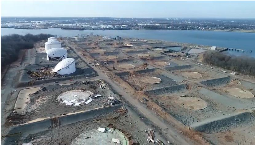
R. Baker & Son recently completed a tank farm demolition project at Port Mobil in Staten Island, New York on the banks of the Arthur Kill. The thirty-eight steel above-ground storage tanks (AST), which had formerly contained a mixture of fuel oil and gasoline, ranged in size from 60 to 135 ft. in diameter and 35 to 60 ft. in height. We were also tasked with abatement and demolition of the facility's administrative buildings.
