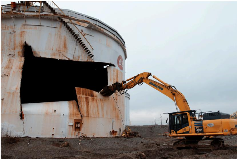
equipped with shears, grapples, and scrapping magnets, as well as several wheel loaders and Bobcat skid steers. Demolition of the tanks entailed cutting the sides into large sections and peeling them away to allow the roof to collapse to the ground, where it was cut into manageable sections for removal. Each week, as many as 80 tractor trailer loads of scrap were transported from the work site to a ferrous metal recycling facility. A total of 12,000 tons were dismantled, removed, and recycled.
