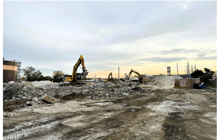
R. Baker and Son recently completed a major demolition project at NRG Energy's Astoria Generating Station in Queens, New York. This complex undertaking involved the removal of three buildings housing twelve Pratt & Whitney twin-pack gas turbine generator sets and their auxiliary mechanical and electrical equipment, as well as two massive oil storage tanks.
