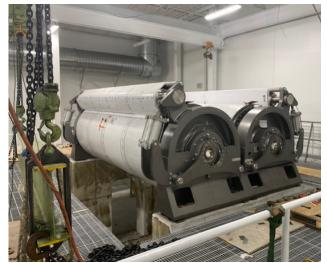
At R Baker, we thrive on challenging projects, and this installation certainly delivered that opportunity. Our client required the rigging, assembly, and installation of four massive 35-ton double drum contact dryers, complete with all accessories. Each dryer would arrive as numerous separate components, presenting a significant logistical puzzle.
