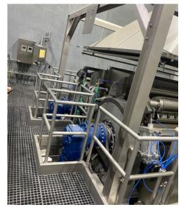
The installation process continued with the attachment of product collection fenders, product augers, large exhaust canopies, end dam assemblies, scrapers, and extensive product piping, actuators, hardware, and hoses.
