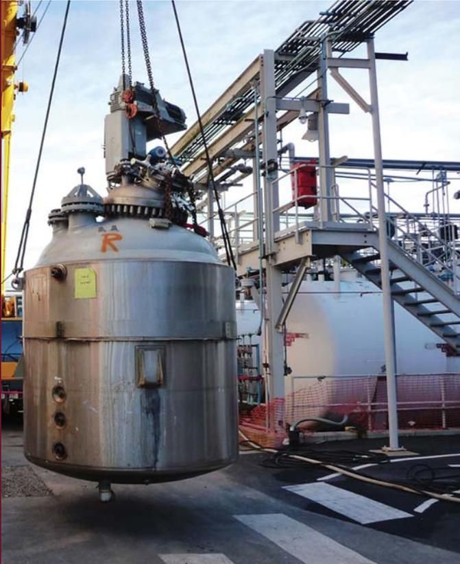
Many details must be taken into consideration when it comes to assembly and reassembly. If equipment is to be disassembled and relocated, it must be pre-determined where equipment will be split, and into how many sections, to prepare for packaging and transport. Every opening along the machine's route through a building – elevators, doorways, windows, roof openings, etc. – must be plotted, because the smallest opening is always the weakest link.
