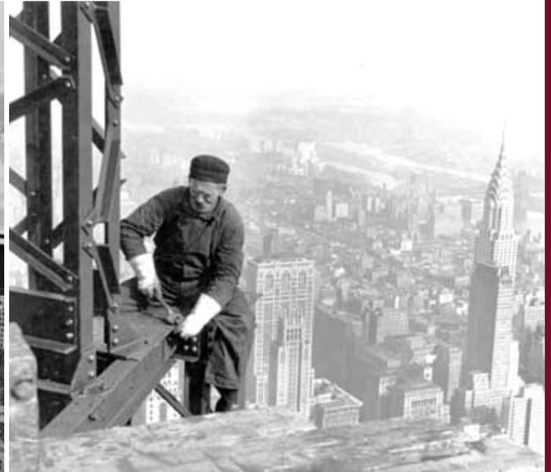
**Construction of the skyscraper was a marvel of efficiency.** Production, transport and construction were choreographed to a science. Steel girders produced in Pittsburgh, PA were erected and riveted in as little as 80 hours from the time they rolled from the furnaces. Roughly 10 million bricks and 200,000 cubic feet of Indiana limestone were used. More than 3,400 workers, including hundreds of Mohawk Indian ironworkers, took part in the project.
